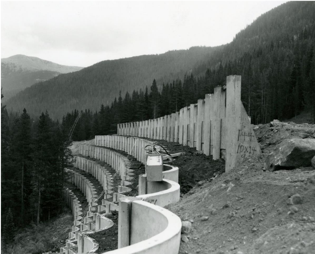
Figure 25. Precast tieback retaining wall, 1975. 127
