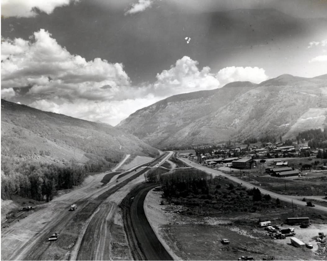
Figure 30. I-70 under construction near Vail Village in the 1970s. 146
